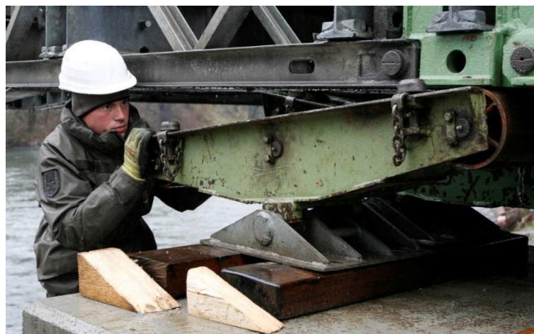
Figure 30: Corrective Maintenance – Temporary repair of a bridge (Bundesheer, Moser, 2009)
